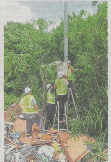
A team from MBI fixing the portable solar CCTV. The cameras cost RM500 each and are set up at hotspots for a three-month period.
