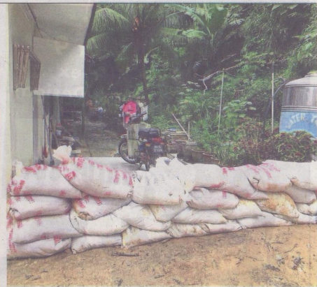
A houseowner in Taman Bukit Teratai, Ampang placed sandbags as a temporary measure to prepare for another mud flood.
