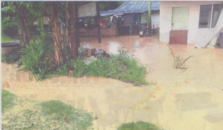
A mud flood in Jalan Bukit Belacan, Lembah Jaya Utara in Ampang earlier this year. — filepics
