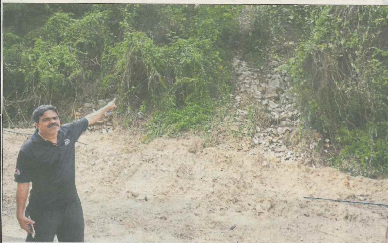
Ganesan showing the site of the mudslide that happened on Jan 23. — Photos: SIA HONG KIAU/The Star
