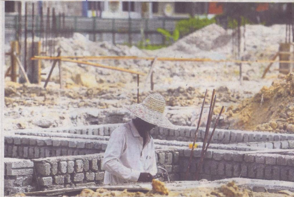
Construction workers have already started work at the site.
