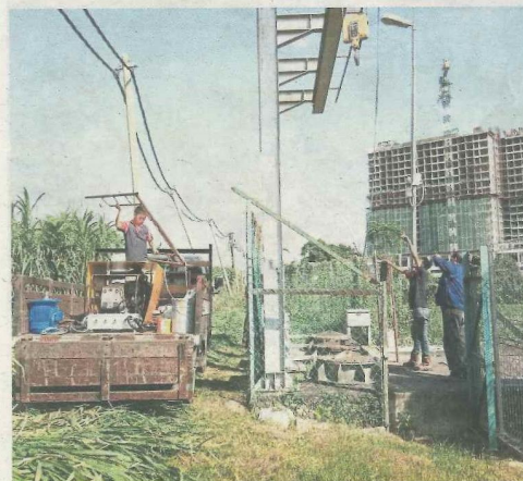
Workers carrying out maintenance work at the Jalan Kebun Bunga, Shah Alam pump house.
