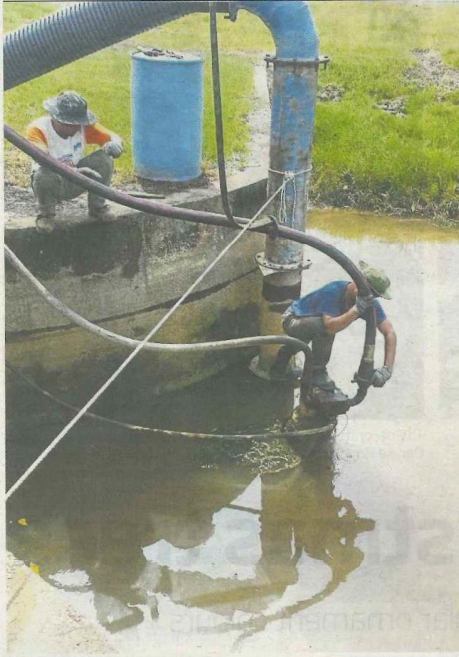
Workers fixing the pipes at Sungai Kembong, Klang as part of the state's flood mitigation programme. — filepic
