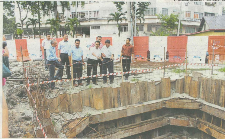
Zaidy (third from right) with members of the Flood Prevention Task Force checking a construction site in Bukit Kuda, Klang under the Ops Lumpur exercise.
