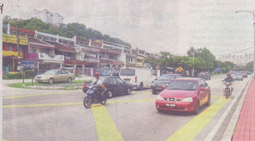
Jalan Mawar is a busy road, making it necessary for MPAJ to build a pedestrian bridge there.
