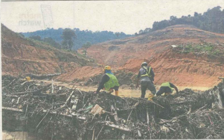
(Top) A downpour caused the retention pond at the SUKE worksite to give way. (Right) SUKE workers cleaning out the culverts after the mud flood.
