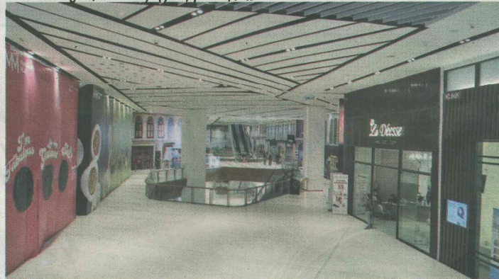
General view of Level 6 in Melawati Mall.
