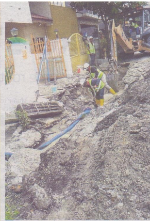
Syabas contractors repairing the burst water pipe in Taman Nirwana 9.
