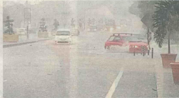
Jalan Bunga Raya in Taman Kencana is often flooded after heavy rain as the drains cannot cope with the volume of water.
