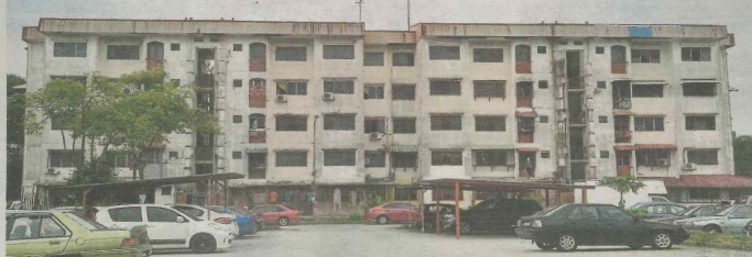
The PKNS flats in Section 24, Shah Alam. PIX BY FAIZ ANUAR
