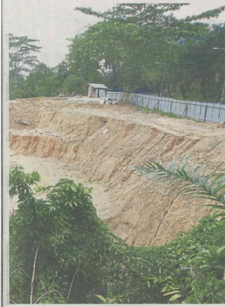
Ukay Heights residents claim that 60,000 tonnes of soil have been dumped at the project site. The loose soil washed down during a downpour affected houses in Taman Ukay Heights.
