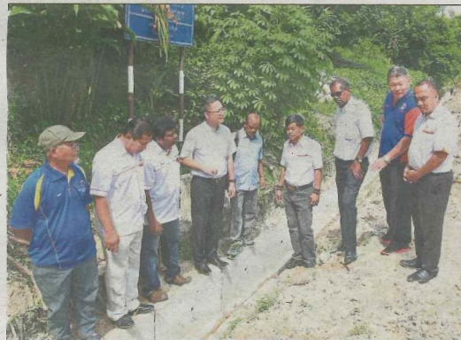
Lai (fourth from left) at the Taman Saga drainage project site in Ampang Jaya, Selangor. With him is Abdul Razak (second from left).
