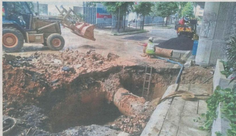
Work in progress: Syabas personnel repairing the burst underground pipe along Jalan Dewan Bahasa in Kuala Lumpur.
