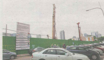
Construction work ongoing at the pocket of open land in Bangsar that was handed over by Bangsar's original developer to the government, then sold to a third party in 2003. — Photos: ART CHEN/The Star
