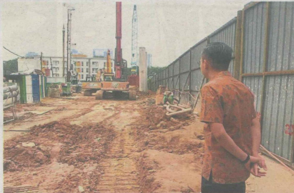
Fahmi visiting the project site in September where he found the contractors working on a Sunday. — Filepic
