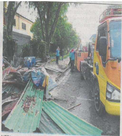
MPSJ personnel demolishing stalls that were built illegally on Jalan Kinrara 2, Puchong.
